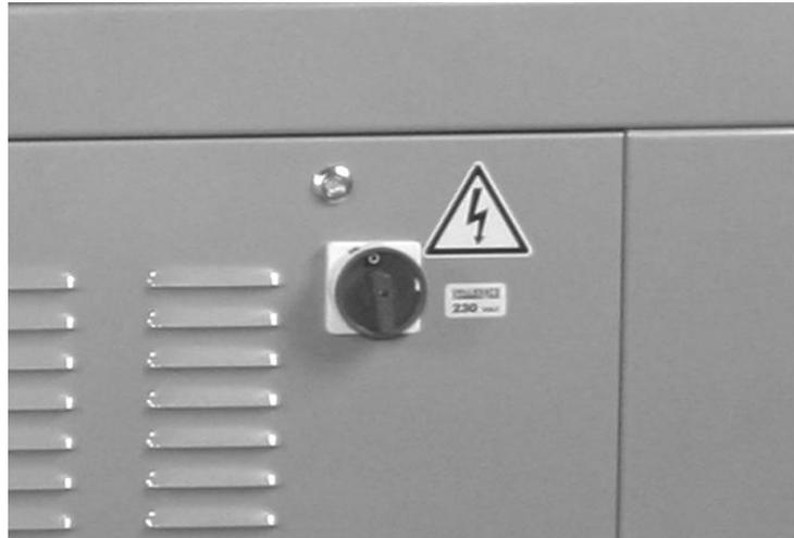
On/off switch is located on front of electrical control panel.
